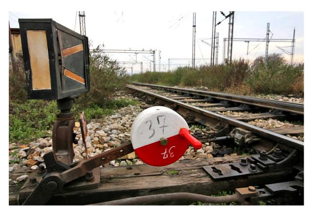
Figure 8. The handrailroad switch, Batajnica, November3, 2020 (Photo: Z. Cvetković)
