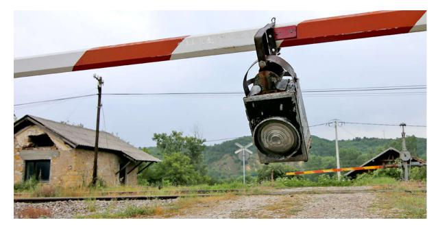
Figure 6. The protected crossing at Čiflik, July 16, 2020 (Photo: Z. Cvetković) The half-barrier and old signallamp
